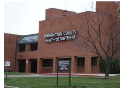
Former Location of Health Monitoring Unit
